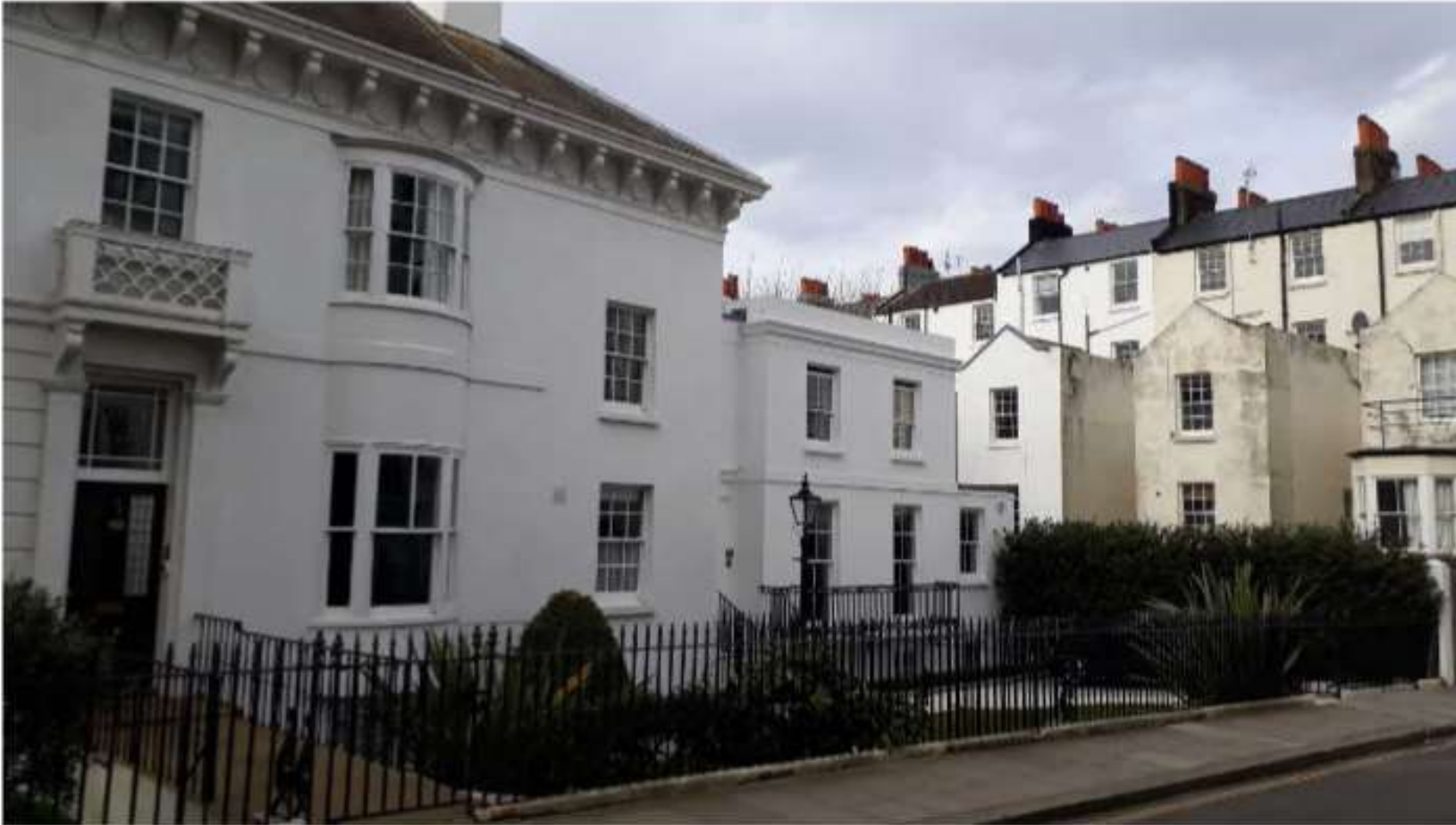
View of site from east on Victoria Road as existing
